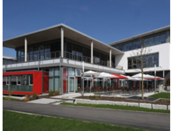
Fig 1: Innovation center at Zwick in Ulm, Gemrany
