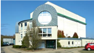
Hattingen, YXLON Inspection Services
